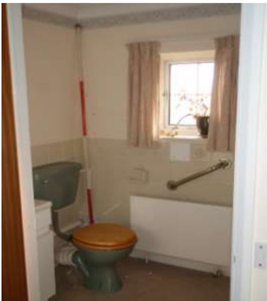
Figure 23 Toilets and Figure 24 hand basins
