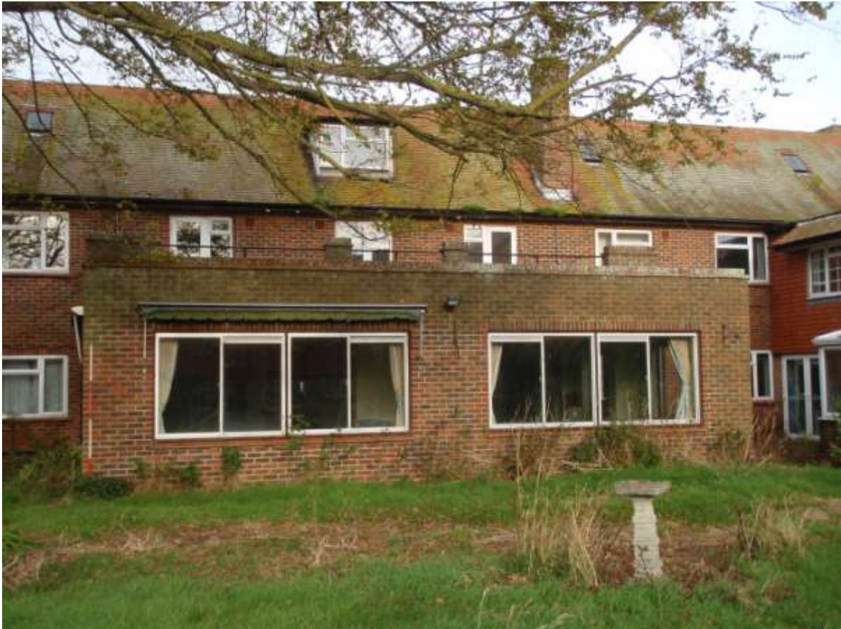
Figure 10 Cheneys south facing facade
