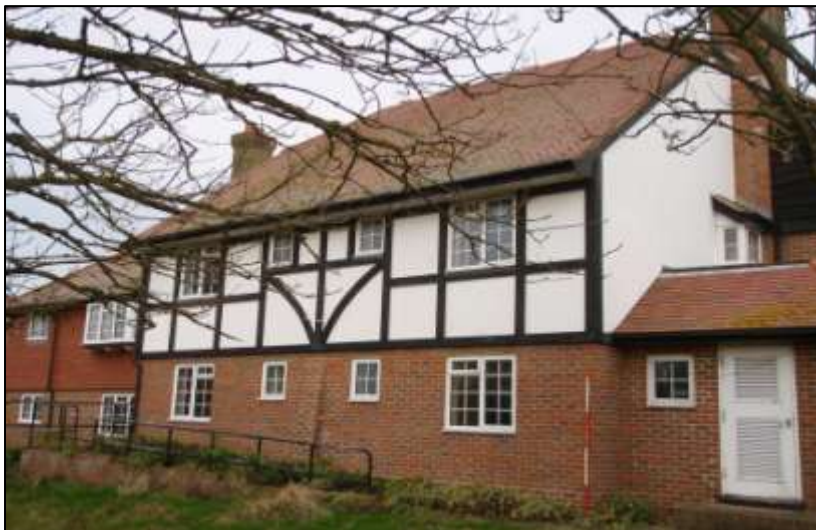
Figure 6. Cheneys extension –looking west
